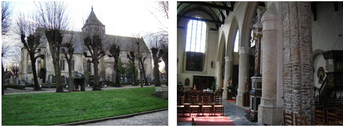
Figure 3.13: 12 th -16 th century church, Wulveringem. Left: Overview photo ( http://nl.wikipedia.org ). Right: Sample 2 is taken at the part of the pillar at the right which is made of ironsandstone.
